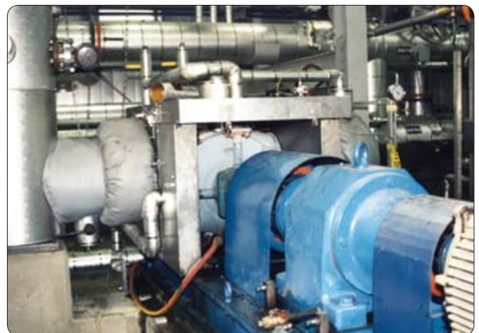
Fully-Jacketed pump in cold climate application
