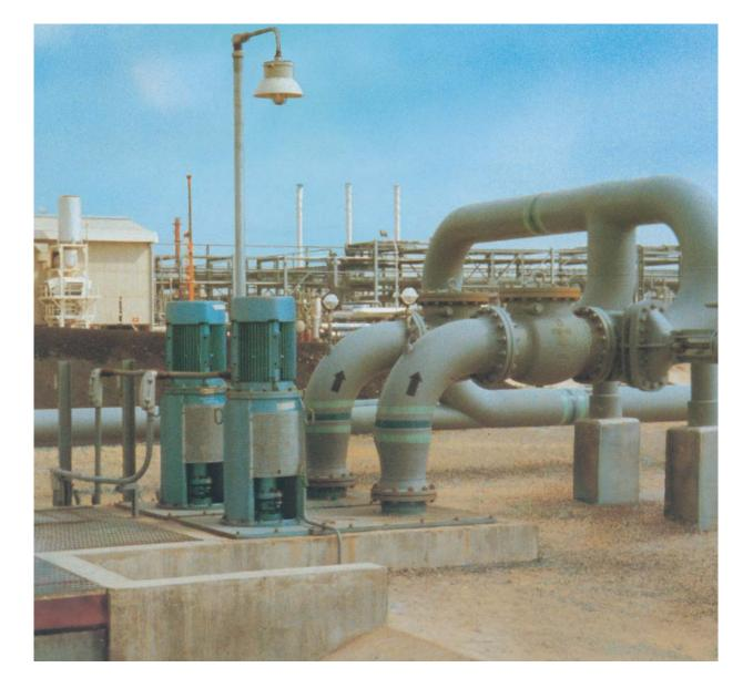
Submersible Long Shaft Pumps for the Chemical Industry Type NCT / NMT
