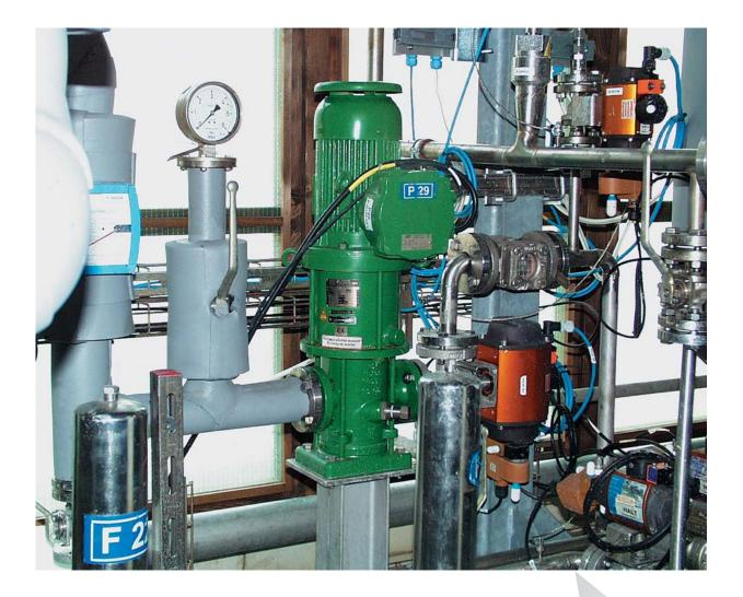
Vertical selfpriming Side-Channel Pumps with magnetic coupling Type SMV our contribution for environmental protection
